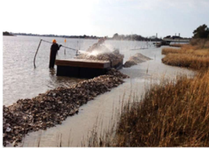
Loose oyster shell sills during construction
